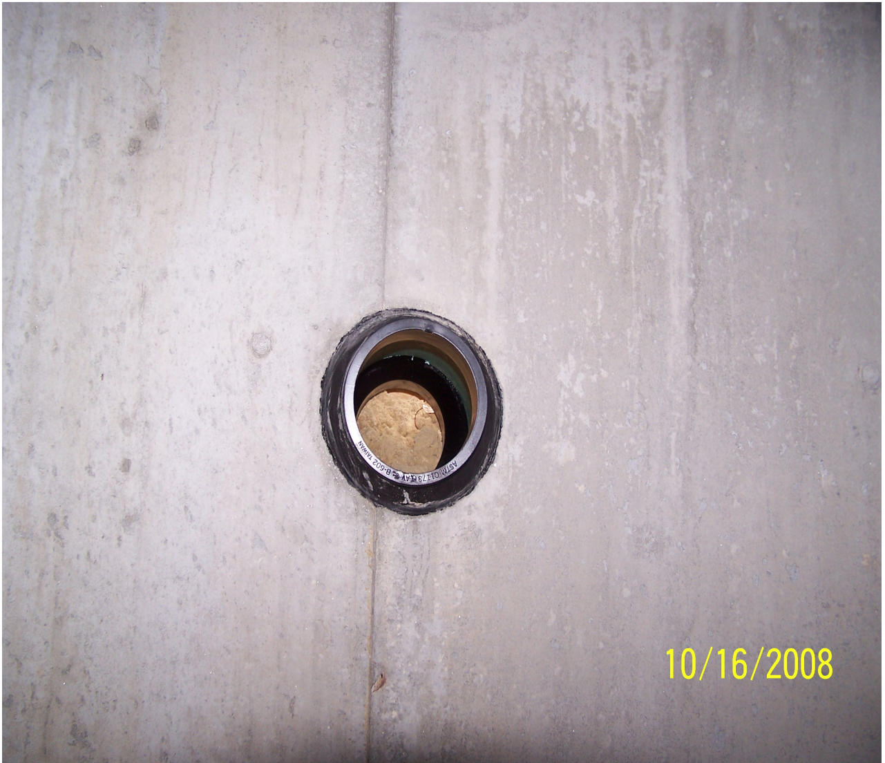
Foundation wall penetration. Requires sleeve and fernco coupling.
