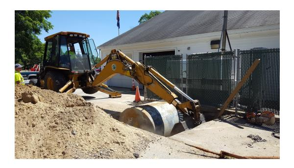
Prepping for the conversion from oil to propane at the Fremont Safety Complex this summer required removal of the buried oil tank. Our talented Highway Department orchestrated the majority of this work.
